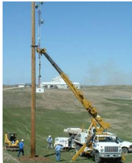
Feeder line from ORC to the Grid
